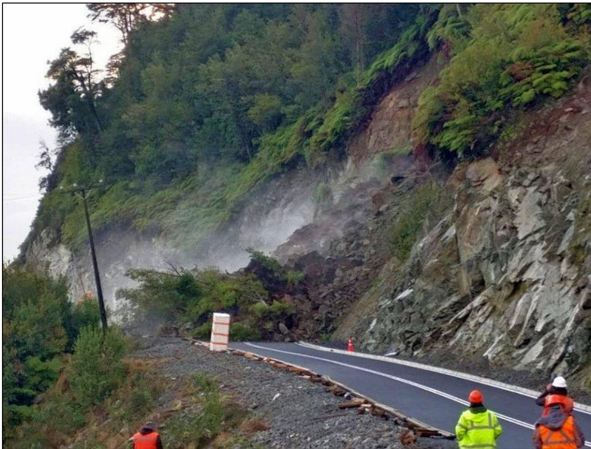
Figure 34 To modernize and pave Route 7, several cuts were made on the slopes of the hill, removing rocks and sediments. This action exposed several outcrops but also generated significant instability on the slopes. The stabilisation of the road may result in the permanent modification of the landscape. For instance, using shotcrete may permanently lose the visibility of some outcrops. Photo: Ruta 7, Chaitén, taken from Diario el Huemul (2018).
