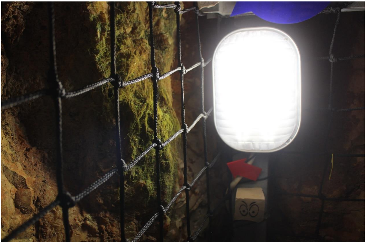
Figure 40 – Lampenflora growth near an incandescent lamp in Pena Cave Interpretive Center placed just to illustrate the consequences of a wrong use of this type of lightning in caves.
